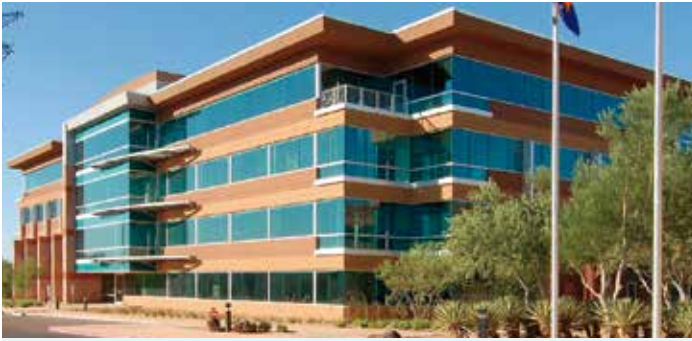
PRINCESS & PERIMETER OFFICE BUILDING 17550 N Perimeter Dr, Scottsdale, AZ
