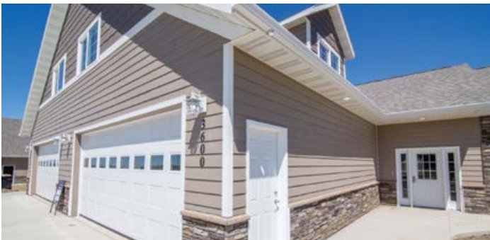
COULEE RIDGE TOWNHOMES 3009 43rd Ave NE, Bismarck, ND
