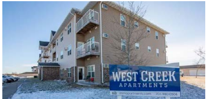
WEST CREEK APARTMENTS 1400 12th St W, West Fargo, ND
